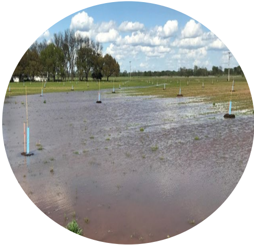
Poor water infiltration
