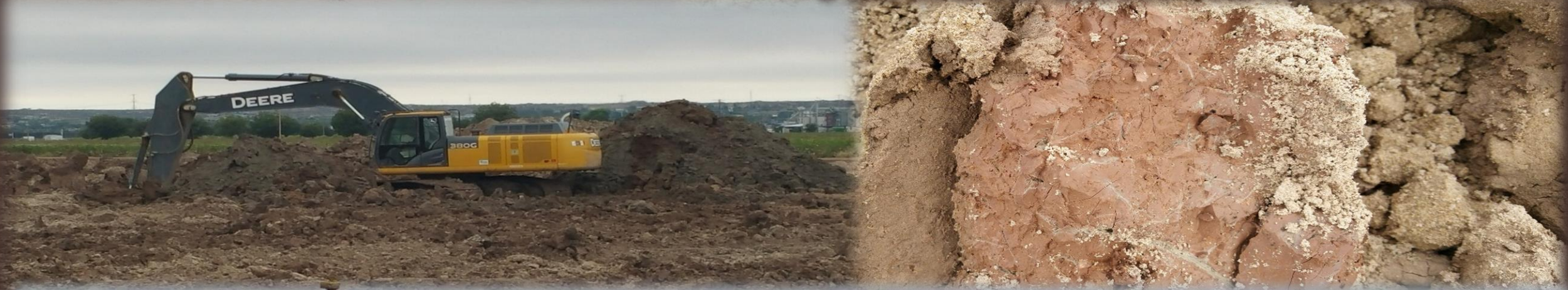
PLOWING WITH TRACKHOE
